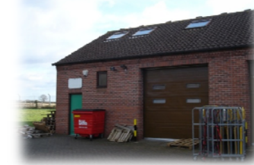
11.1. Light Industry Small Unit on Tattershall Road
