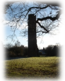
5.14. Tower on the Moor
