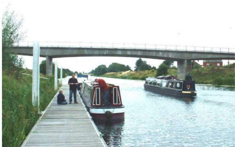
Moorings at Kirkstead Bridge
