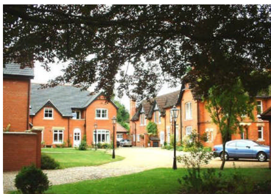
Renovation of previous school dormitories
